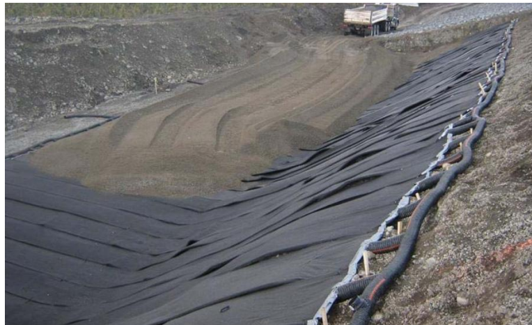
Figure 4. Geocomposite sheet connected to drainage pipes at top of embankment [9].
