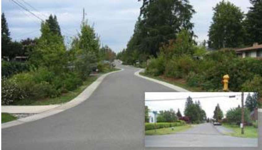
Figure 6. Before and after photo of SEA project [12].
