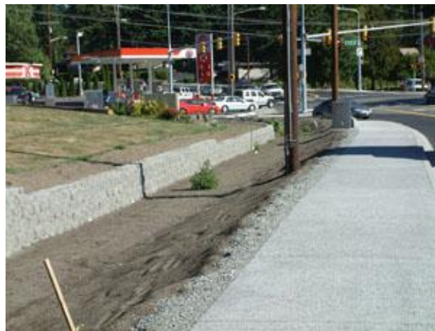
Figure 7. Completed LID Project [14].
