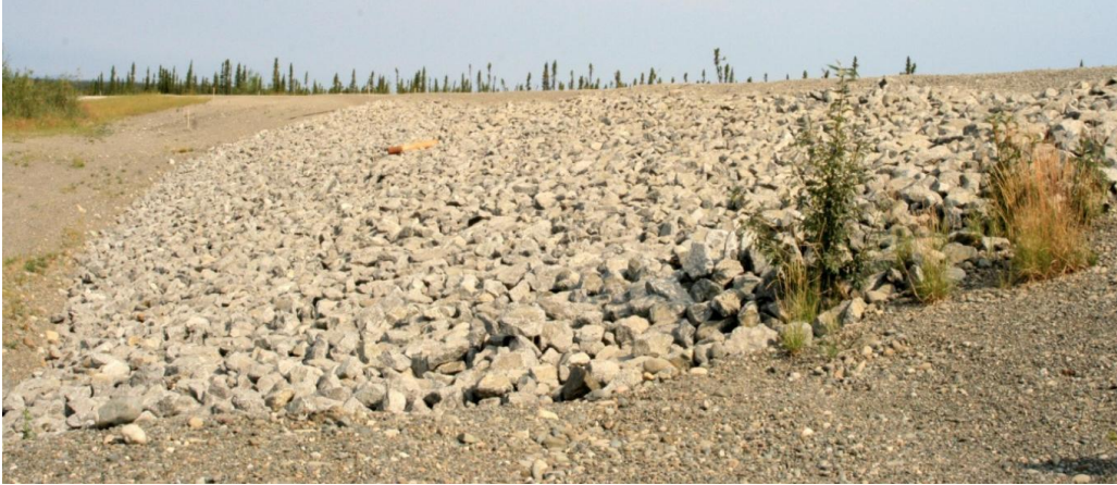
Figure 3. Uncovered air cool embankment showing rock material used for construction [8].
