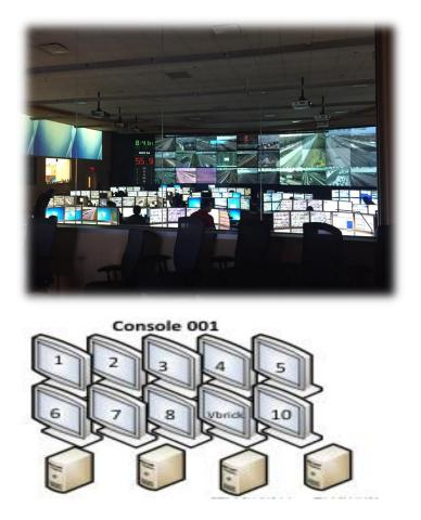
b. Operators had a large quantity of computer screens and workstations. Each operator had about ten screens; which I learned, were operated through a KVM Switch (a device that allows switching the mouse and keyboard from computer to computer).
