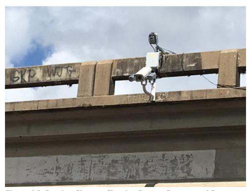
Figure 4-8: Bracket Close-up Showing Sensor, Camera, and Processor
